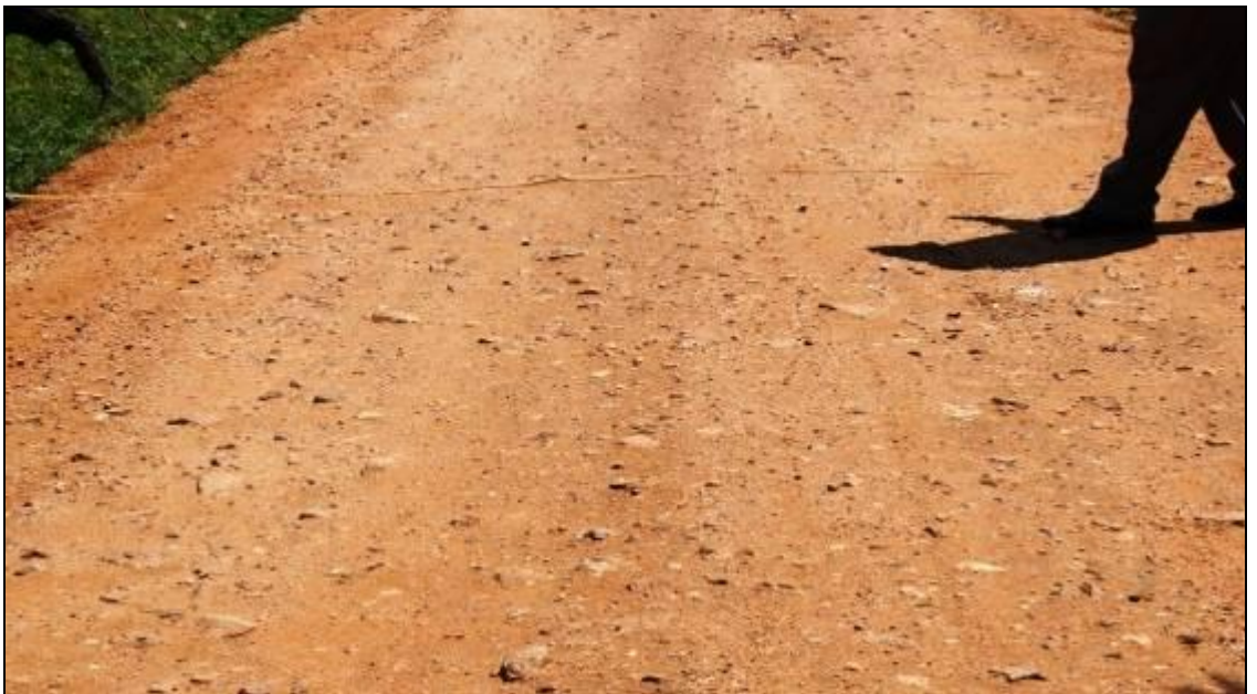
Picture 24: A section on Katooke –Kagadi Road with inferior sub-grade that did not allow proper bonding, causing poor riding quality due to stoniness.
