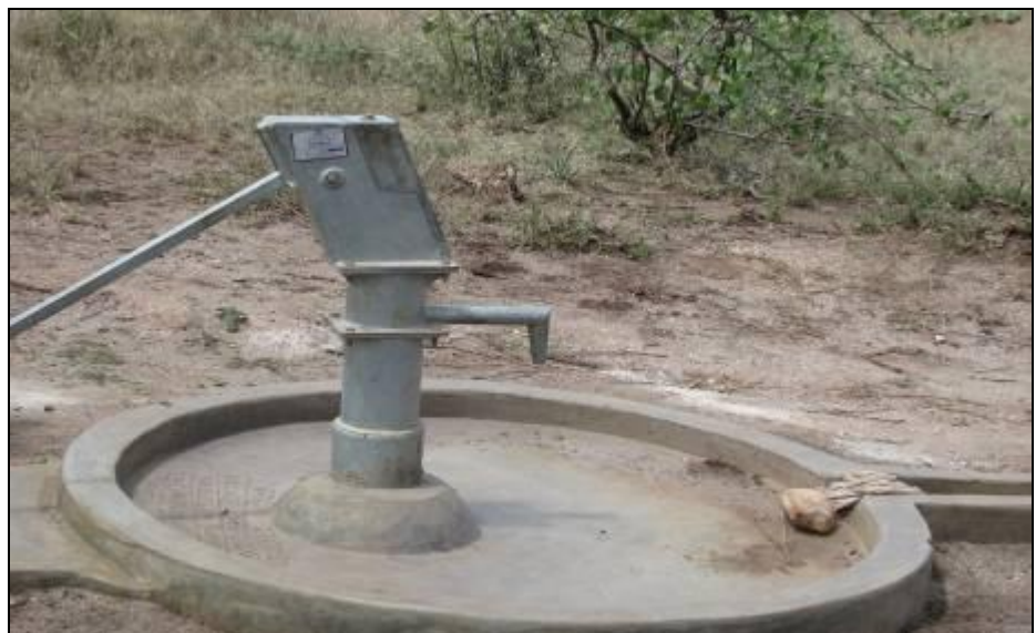
Picture 9: A borehole constructed in the financial year 2009/2010 found dry barely four months after construction and before hand over.
