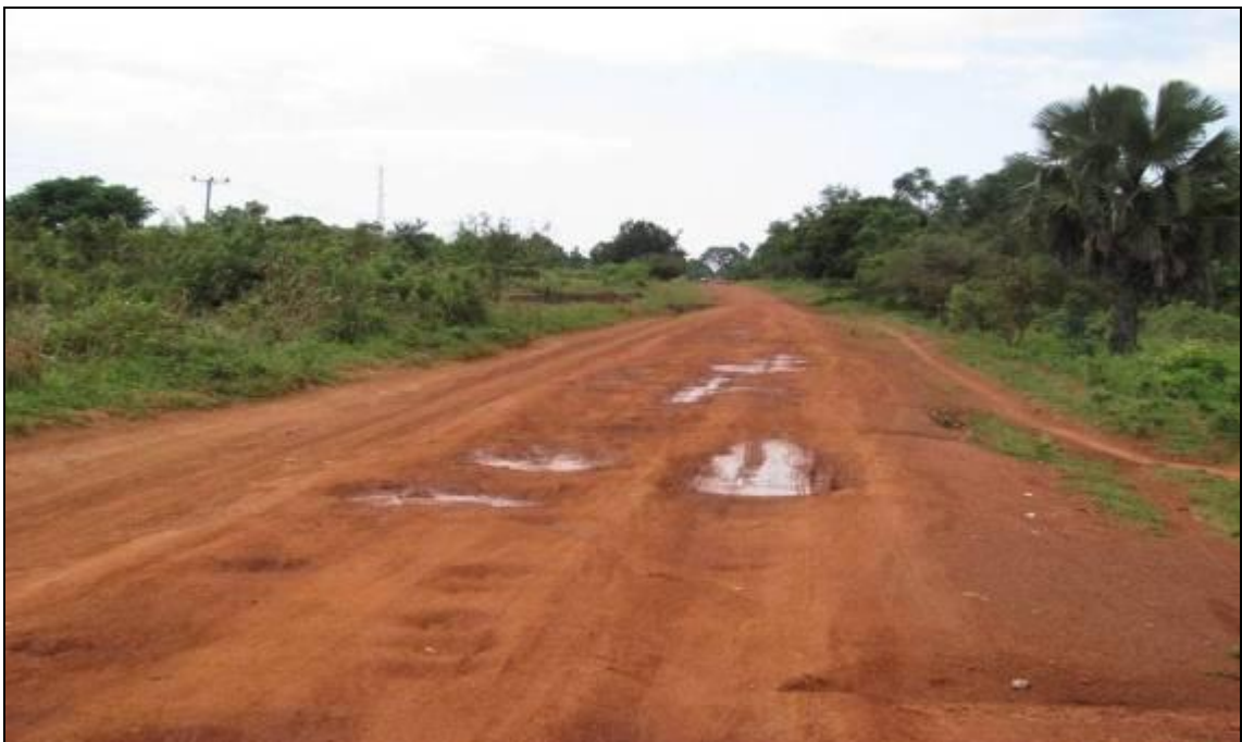
Picture 21: A section of Ngetta Puranga from Km 2+00 to 27 where the entire carriage way has potholes and rutting.
