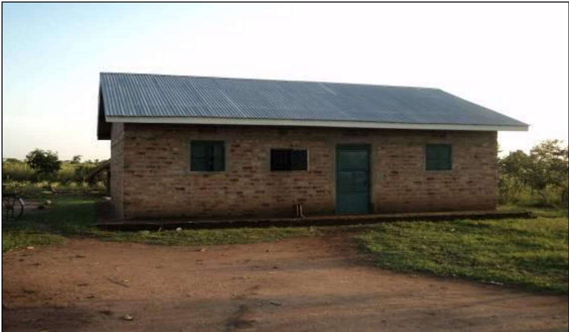
Picture of a newly constructed house of a member of Ongica Beekeepers Association (OBA), in Lira District, taken on 11 th Nov 2010
