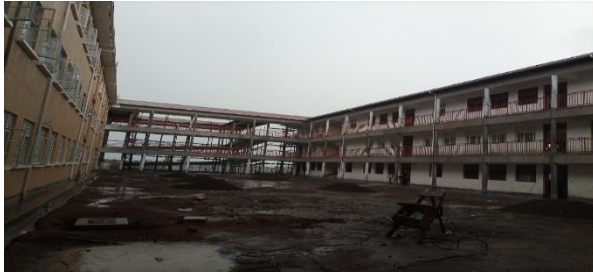
Buildings (construction in progress) Faculty of Education
