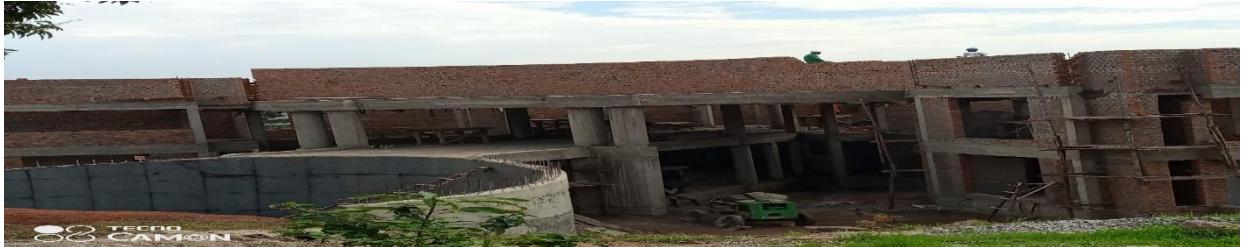
Main Administration at Entebbe under Construction
