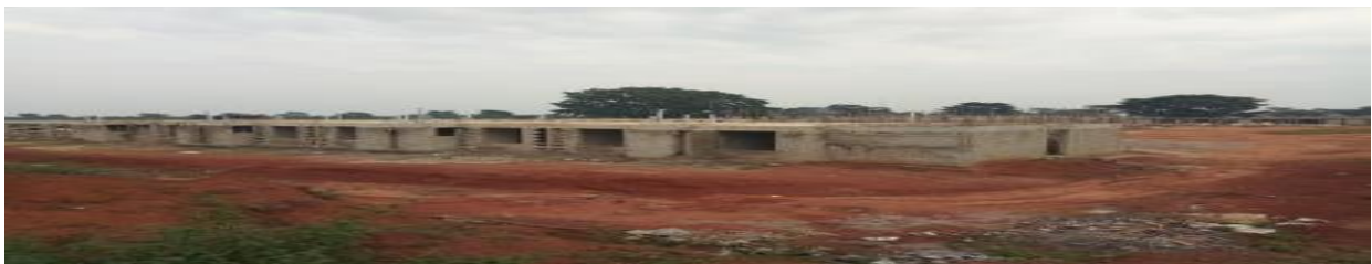
Construction of Hostel at Kasolwe Stock Farm by Jofa Associates
